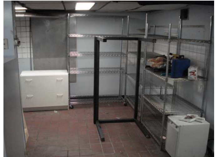
Lower Level Kitchen
